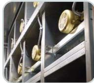
FANWALL provides superior reliability as a result of its built-in redundancy. If one fan fails, only that portion of the airflow is lost, unlike
