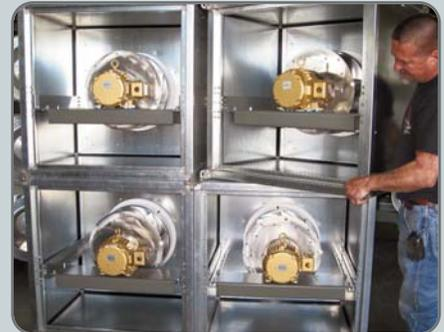
Stack FANWALL cells in a fraction of the old fan footprint to form a FANWALL array of any dimension.
